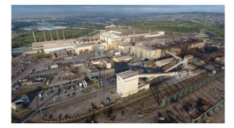
Includes primary and secondary EAF steelmaking, vacuum degassing, ingot casting, continuous casting, bar and coil rolling, and bar processing & inspection.
